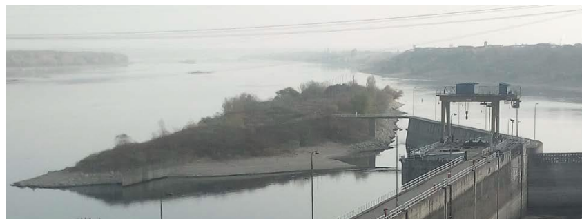
Figure 4.2 - Embankment on the river side in the downstream berthing area at HPNS "Djerdap 2"
