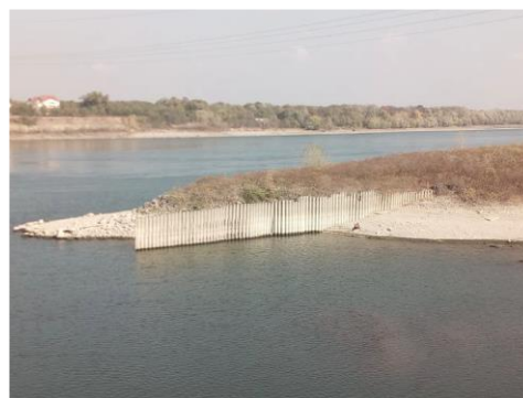
Figure 4.3 - Upstream spike of the embankment on the river side of the downstream berthing area at HPNS "Djerdap 2"
